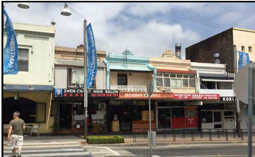
Figure 6 Adjoining development to the south (No 158-166 Norton Street)
