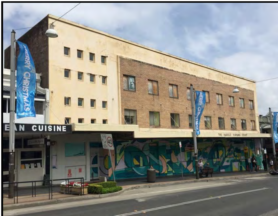
Figure 4 Existing Development on the site from Norton Street
