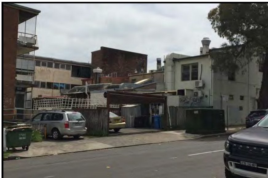
Figure 7 Adjoining Development to the South (rear of No 158-166 Norton Street) - Carlisle Street elevations
