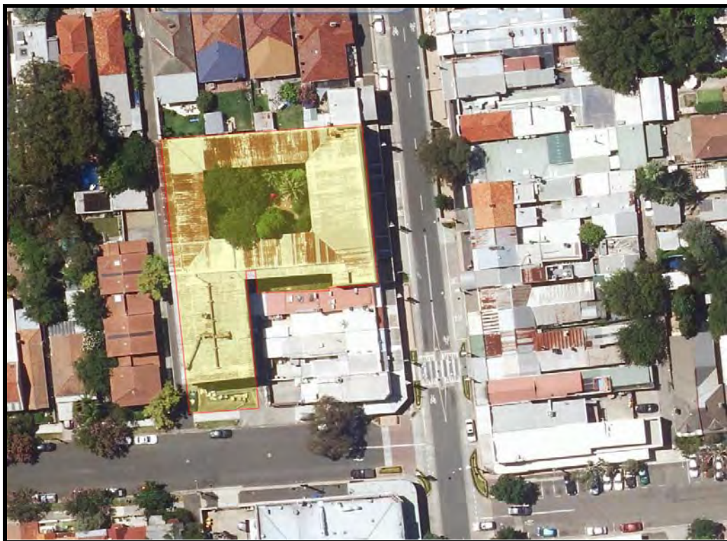
Figure 3 Site Location (Source: SIX Maps)
